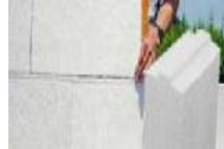
Gaz beton duvar
